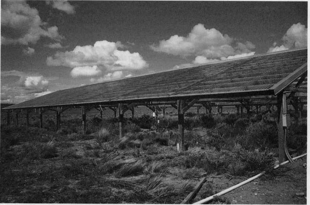
Figure 1. Fixed location rain shelter. Both this picture and the one in Fig. 2 were taken after the Dynaglass® glazing had been installed.
